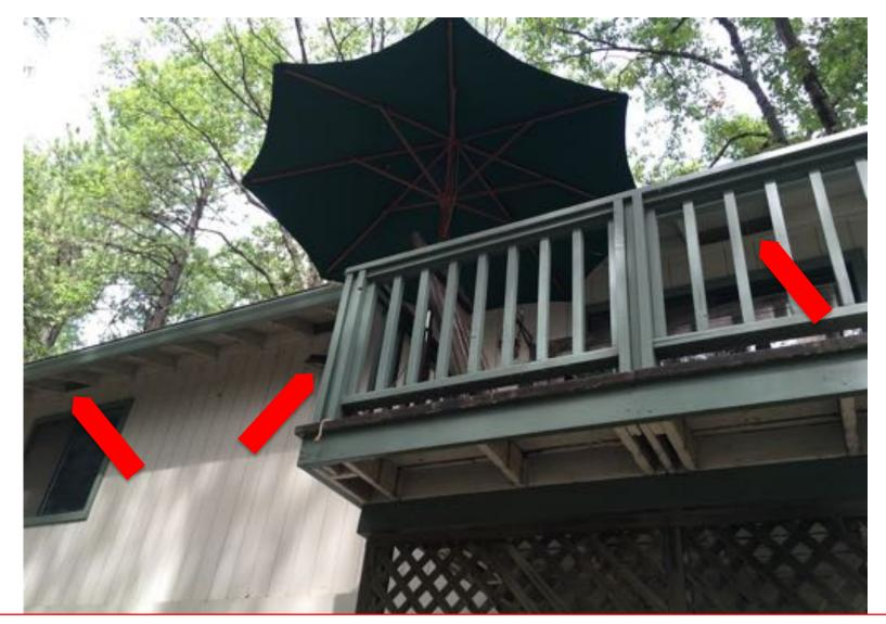
Arrows show attic vents which already had 1/8". Redwood lattice (bottom) was very old and dry and has been replaced with plastic lattice. We will box in underneath the deck surface.
