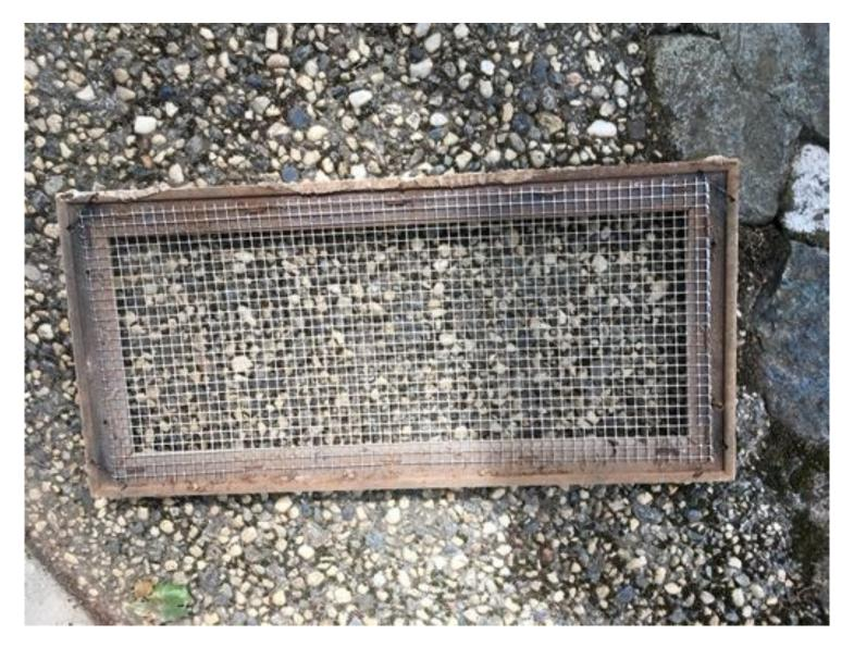
Decided to attach 1/8" hardware cloth (stores don't call it "screening") inside each foundation vent with a staple gun, then just re-attach.
